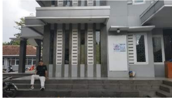
Gambar 4.5. existing akses masuk masjid At-taqwa
