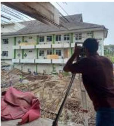
Gambar 7. Penentuan As Pile Cap
