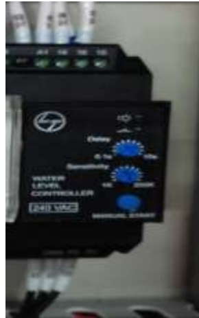
Gambar 4. Water level control
