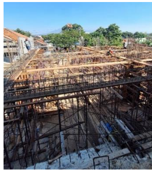
Gambar.2 Bekisting Balok
