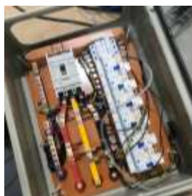
Gambar 3. Hasil Wiring RCBO
