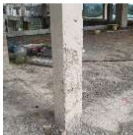
Gambar 1. Kolom Cacat ( honeycomb )
