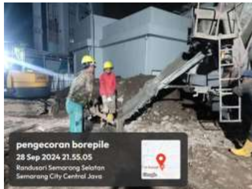
Gambar 2. Pengecoran Bore Pile
