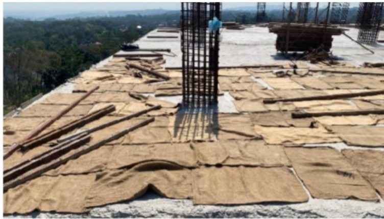
Gambar 14 Perawatan Beton ( Curing )
